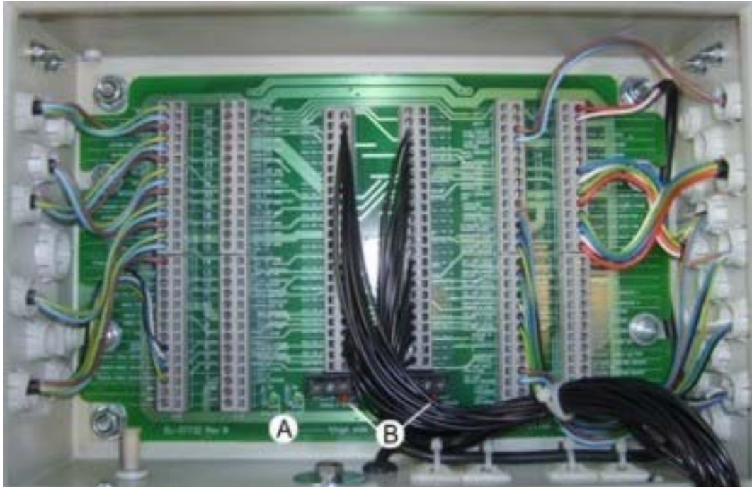
SB361 and SB401 F and R junction boxes (above)
